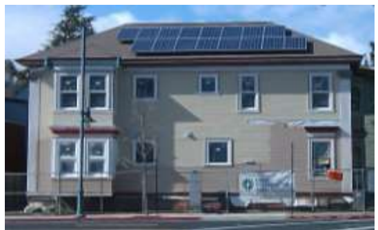
Magnolia Terrace under construction, March 2011
